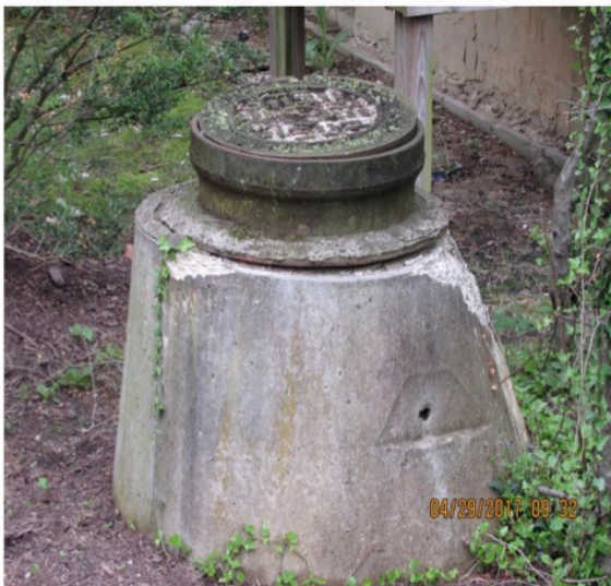
photo 3 (not on map) (May 16, 2017 replaced blurred picture of broken frame base flange on Manhole 20756)
