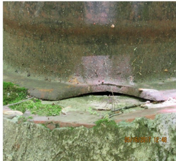
photo 3 (not on map) (May 16, 2017 replaced blurred picture of broken frame base flange on Manhole 20756)
