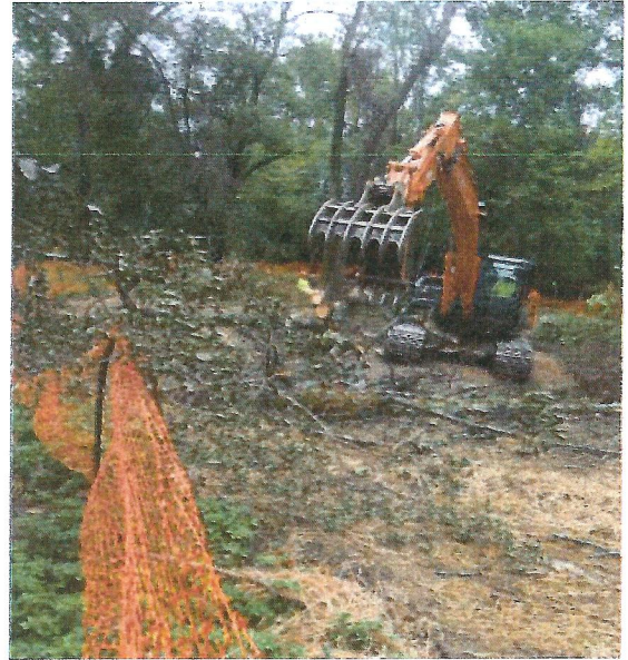
A bulldozer clears trees along Roland Run.
