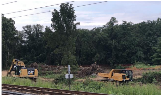
Figure 2: Construction of Roland Run Stream Restoration Project.
